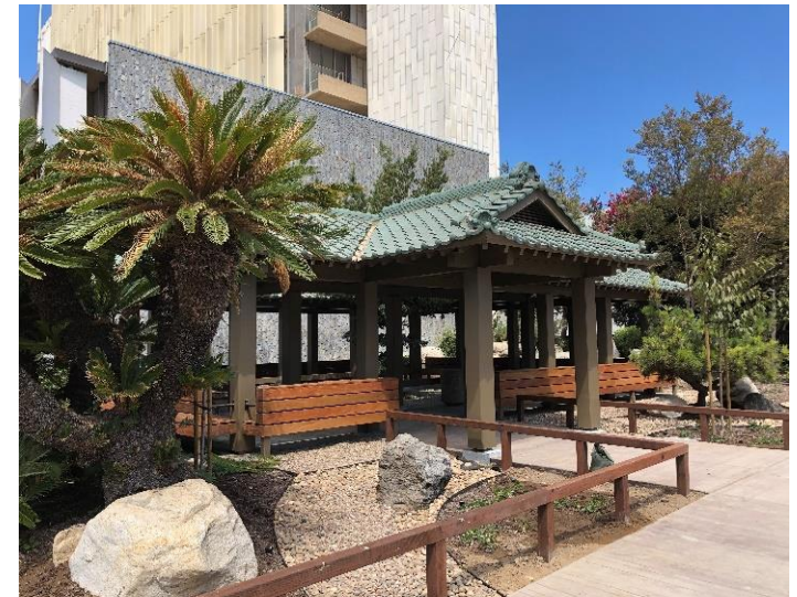
Civic Center Improvements: Pavilion Renovation
