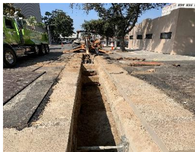
Bush Street Water Main Improvements
