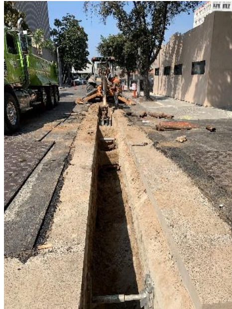
Bush St. Water Main Improvements
