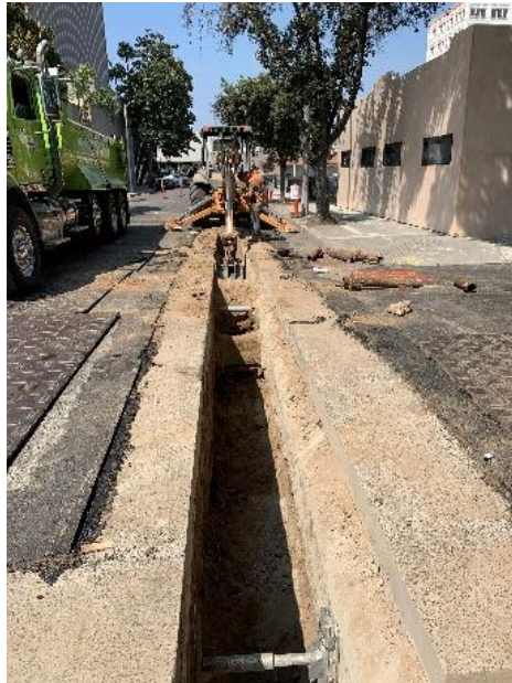
Bush St. Water Main Improvements
