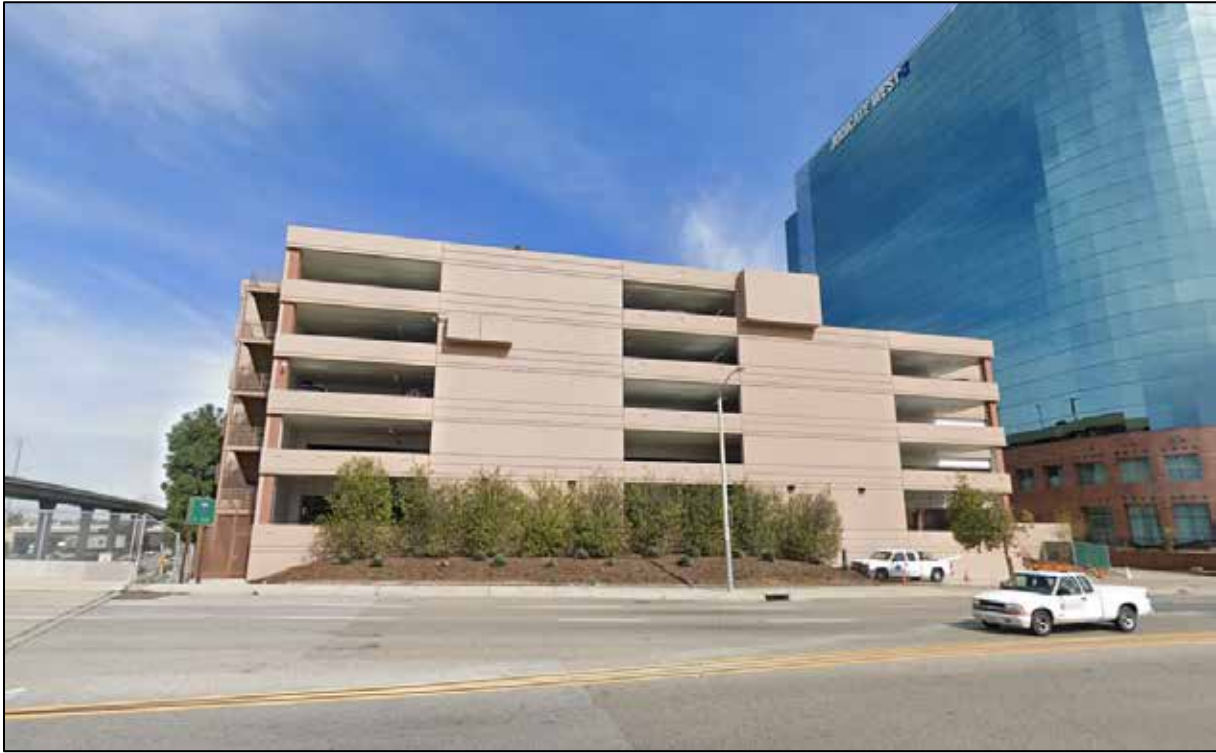
1851 East First Street – antennas mounted onto the wall
