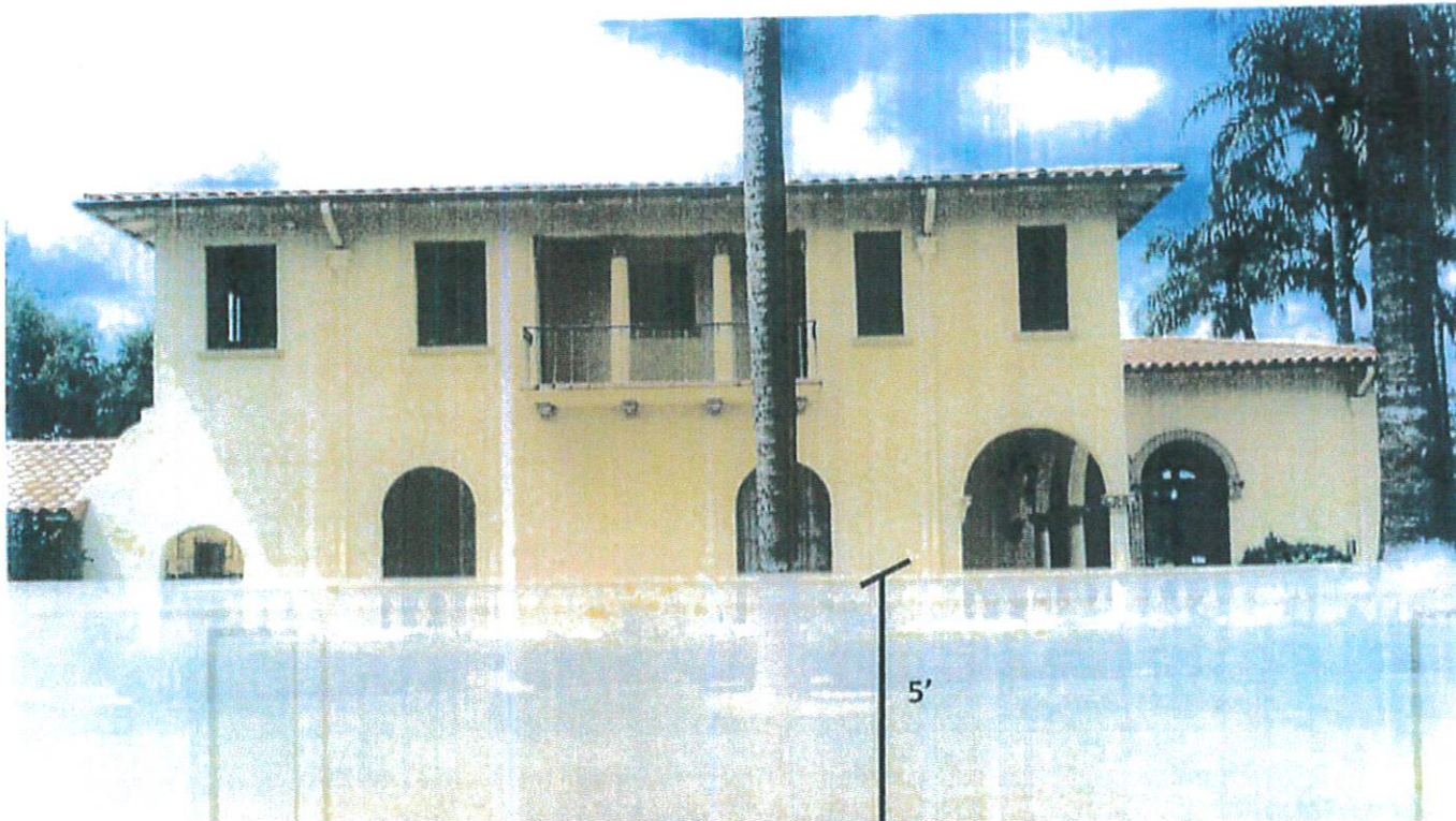
View with 5 ft. wall
