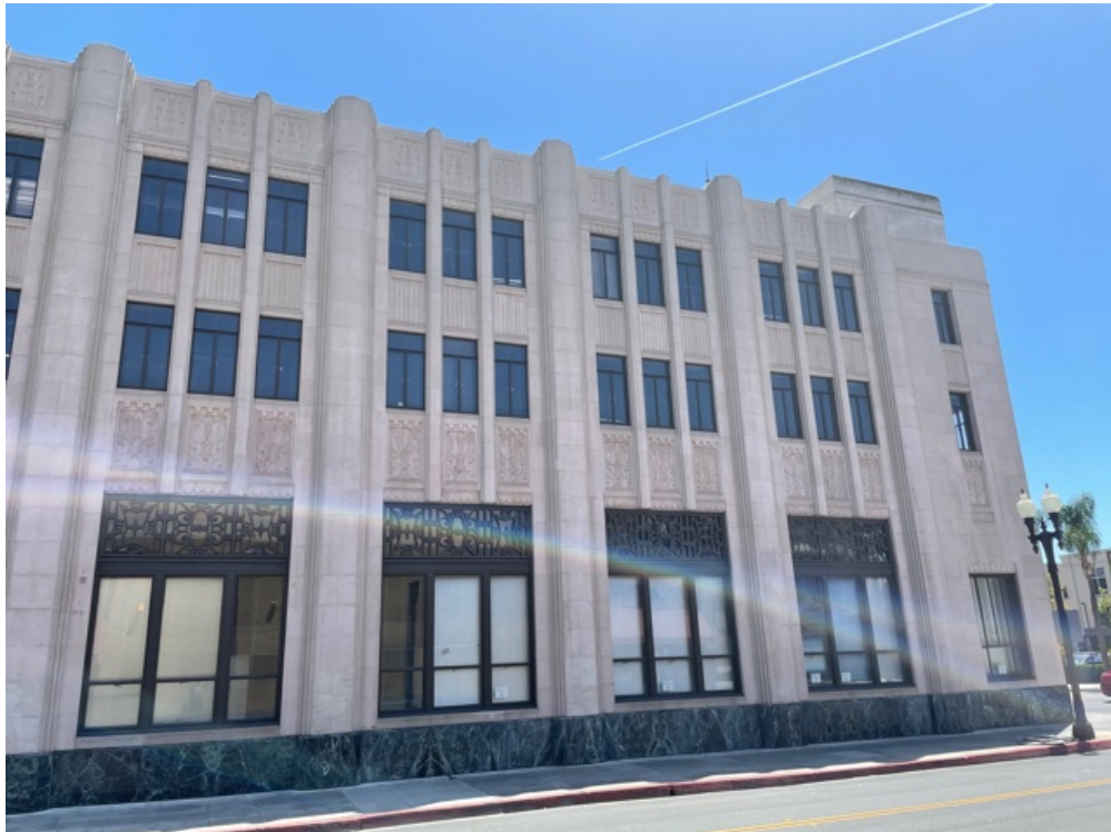
HPPA-2021-19 OLD SANTA ANA CITY HALL 217 NORTH MAIN STREET SITE PHOTOS
