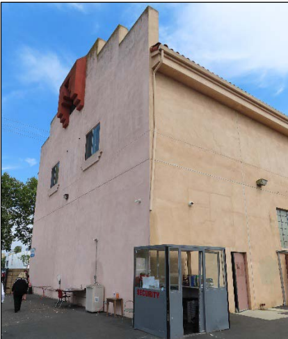
View southeast of the north façade, two-story wing.
