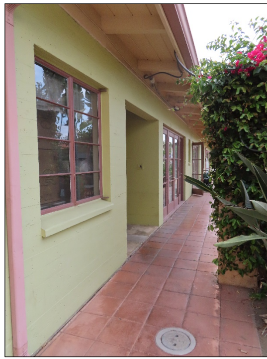
View west of the north façade, one-story wing.
