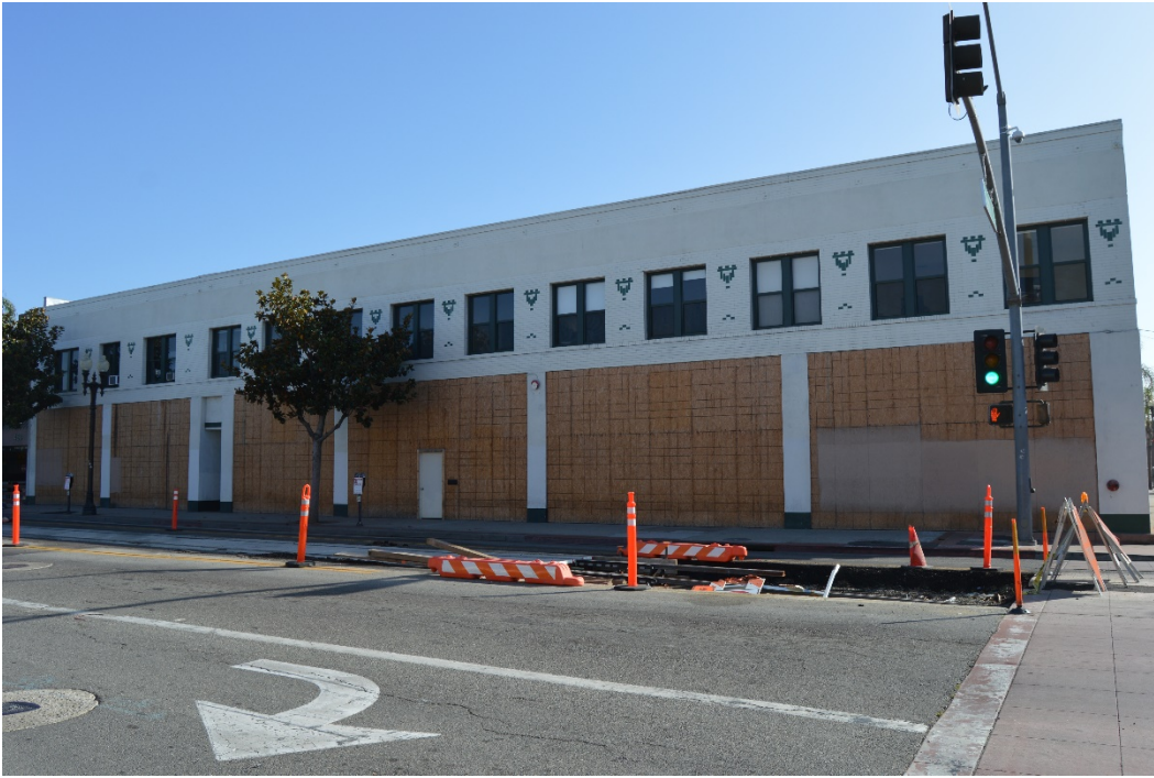
North façade, view facing southeast.
