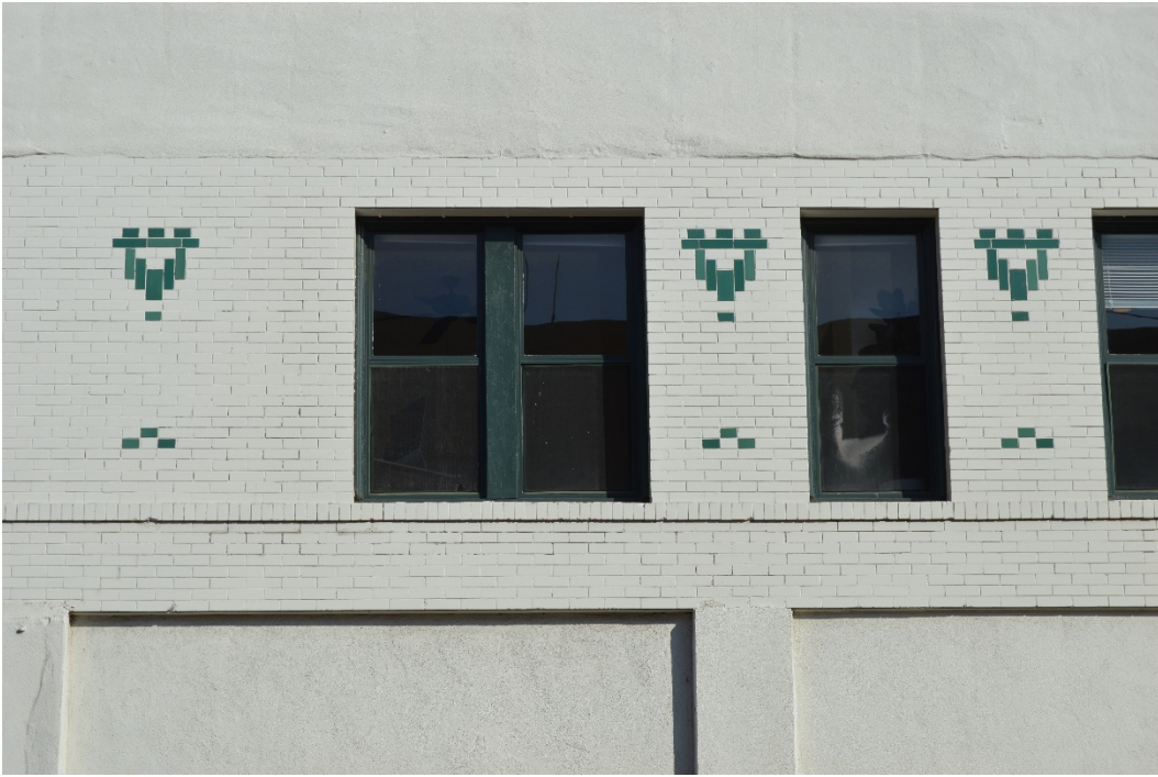
West façade with detail of glazed brick cladding, view facing east.
