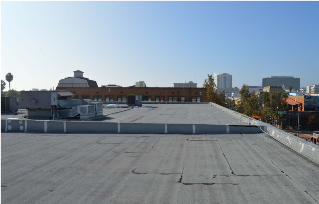
Existing condition on roof, view facing west.
