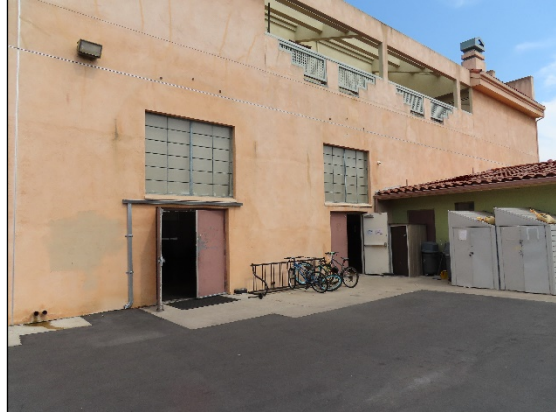
View southeast of the west façade of the two-story wing. Note the 1980s addition.
