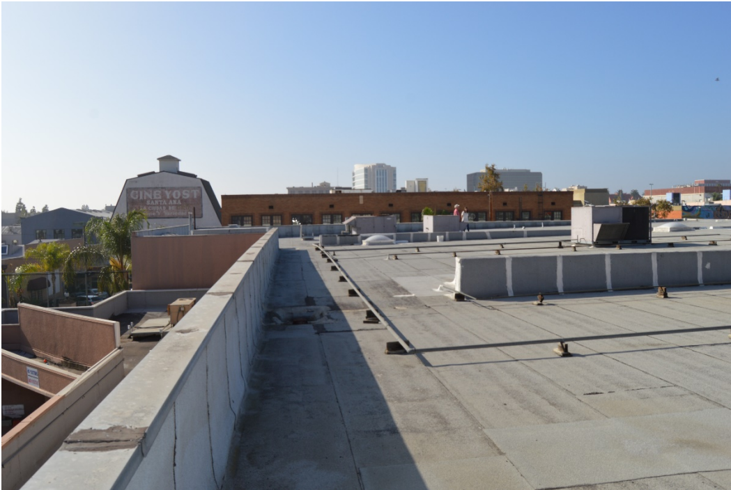
Existing condition on roof, view facing west.
