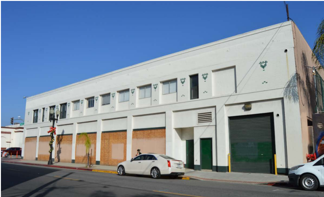
West façade with infilled window bays, view facing northeast.
