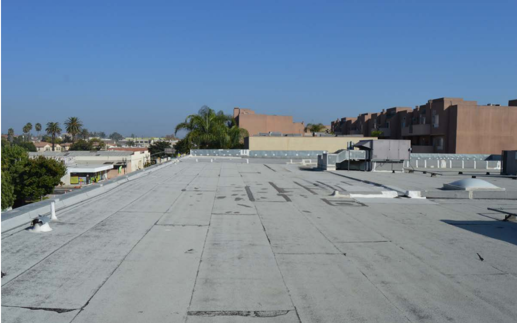
Existing condition on roof, view facing east.
