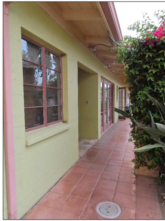
View west of the north façade.
