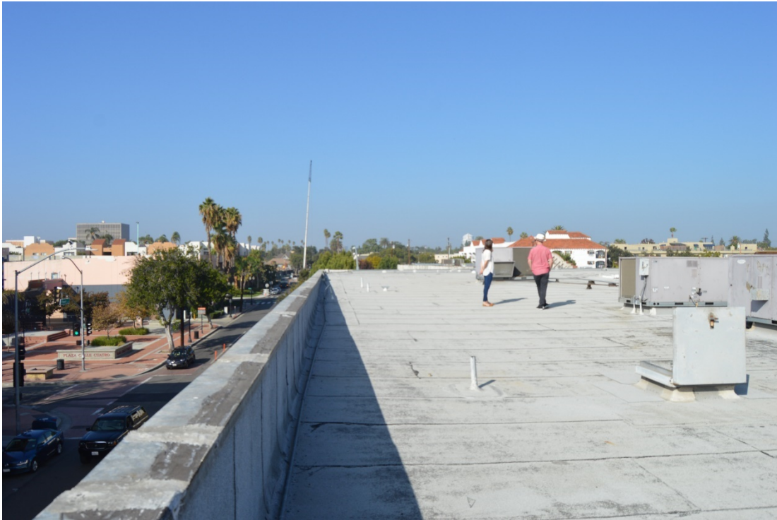
Existing condition on roof, view facing north.
