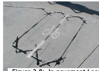
Figure 2.8: In-pavement Loop Detector
