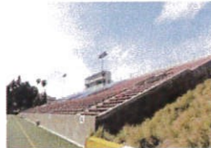
Santa Ana Stadium Structural Improvement
