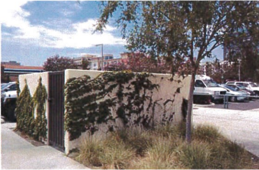
Trash and recycling enclosures should use the same materials as the primary building and screen the area employing elements such as solid masonry walls, berms, and landscaping.
