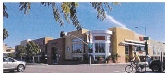
Special attention should be paid to corner features of buildings at prominent intersections.
